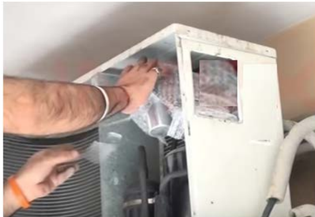
Fig. 5.5.14: Covering the connection box
