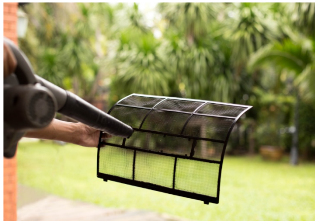
Fig. 5.5.5: Washing the filter
