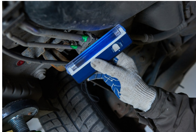
Fig 4.10.16: Leak detection using ultra-violet lamp
