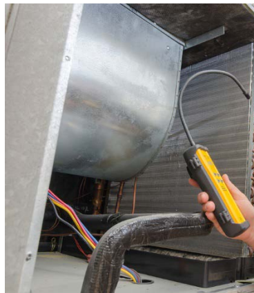
Fig 4.10.17: Leak detection using electronic refrigerant detector
