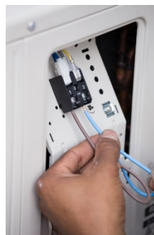
Fig. 5.4.20: Connecting electric wires
