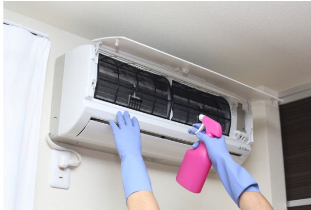
Fig. 5.5.4: Cleaning the dust
