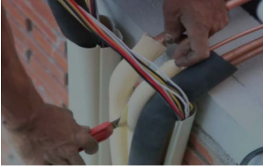
Fig. 5.4.23: Wrap piping joints with insulating tape
