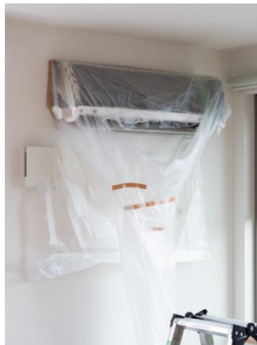
Fig. 5.5.8 Hanging the wash bag around the indoor unit
