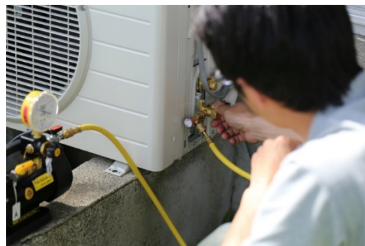
Fig. 5.4.22: Remove air and humidity
