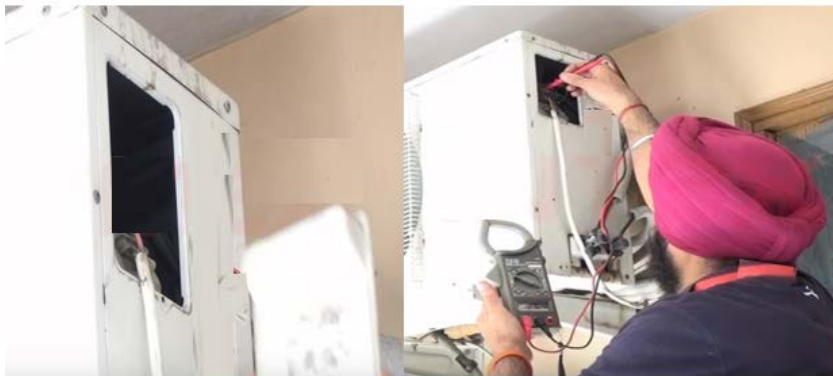
Fig. 5.5.11: Measuring voltage and current
