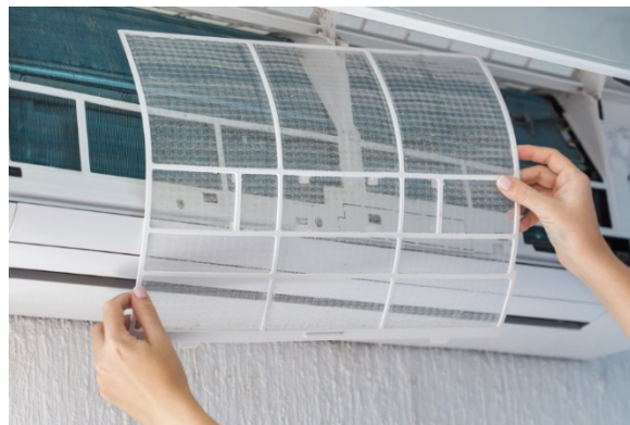
Fig. 5.5.3: Taking the filter out
