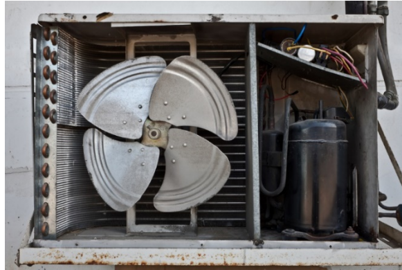
Fig. 5.5.13: Parts of outside unit
