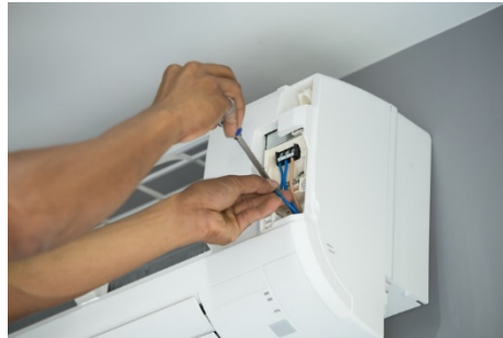
Fig. 5.5.7: Remove the front cabinet
