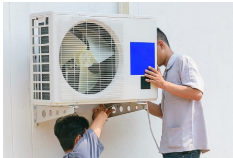
Fig. 5.4.19: Outdoor unit location
