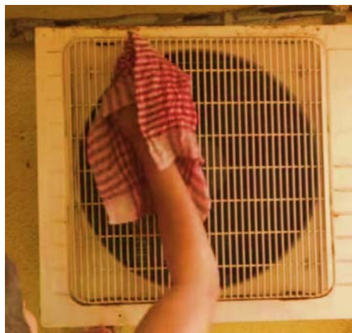
Fig. 5.5.6: Cleaning of outdoor unit
