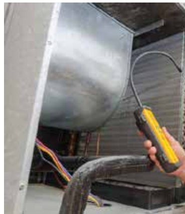
Fig. 4.2.17: Leak detection using electronic refrigerant detector
