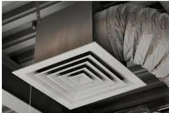
Fig 7.1.4: Exposure of air diffuser
