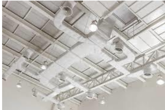
Fig. 7.1.5: Exposure of ductwork
