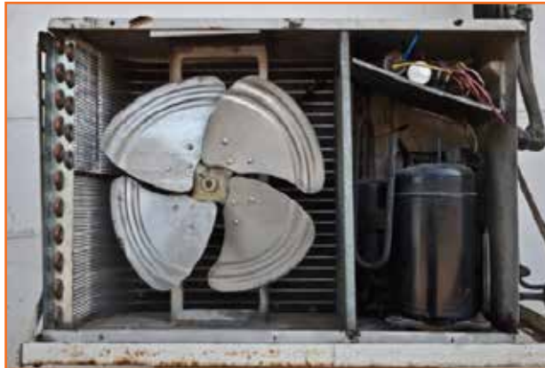
Fig 5.3.36 Parts of outside unit
