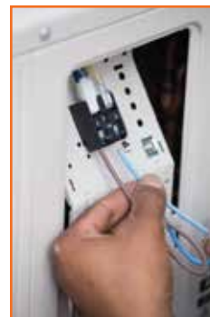
Fig 5.3.17 Connecting electric wires
