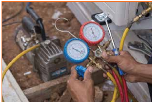
Fig 5.3.35 Measuring pressure using manifold gauge
