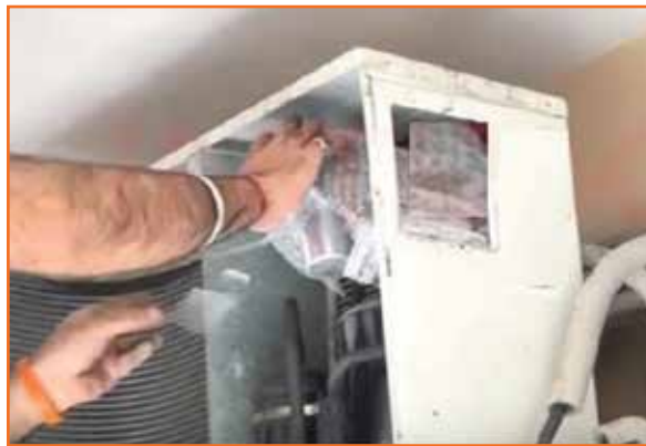
Fig 5.3.37 Covering the connection box
