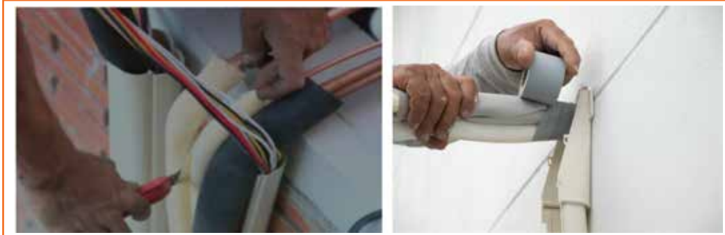
Fig 5.3.20 Wrap piping joints with insulating tape
