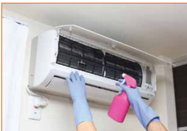
Fig 5.3.27 Cleaning the dust
