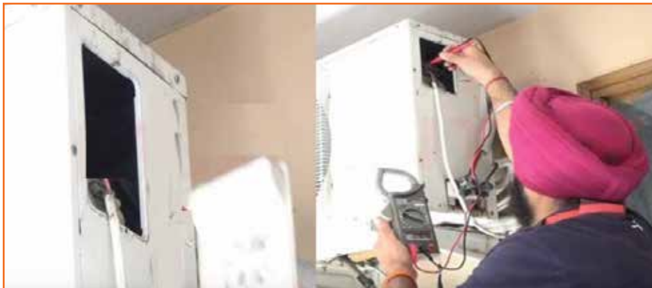
Fig 5.3.34 Measuring voltage and current
