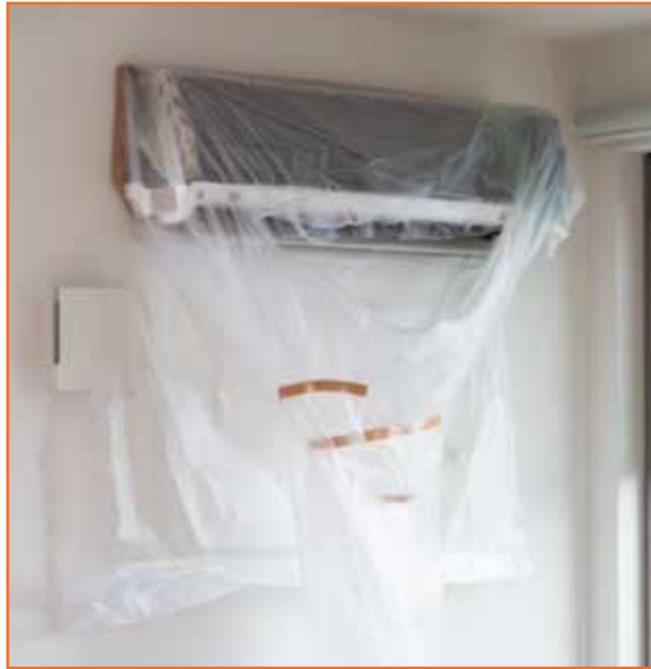
Fig 5.3.31 Hanging the wash bag around the indoor unit
