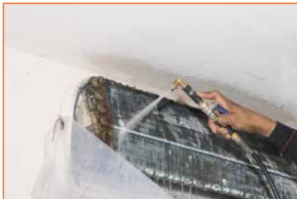
Fig 5.3.32 Cleaning the indoor unit
