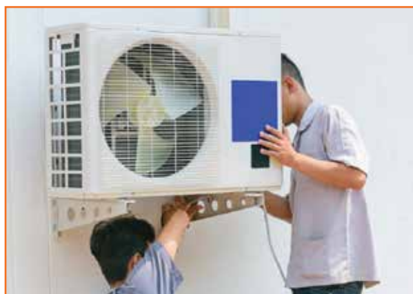
Fig 5.3.16 Outdoor unit location
