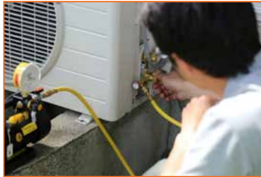
Fig 5.3.19 Remove air and humidity
