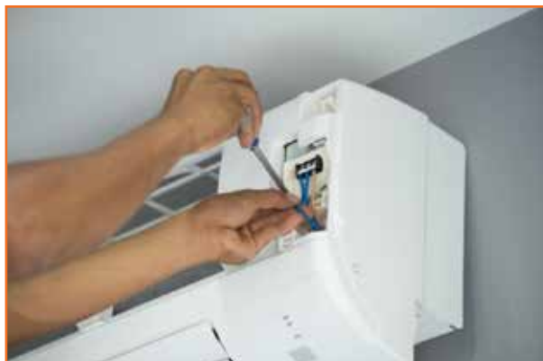
Fig 5.3.30 Remove the front cabinet
