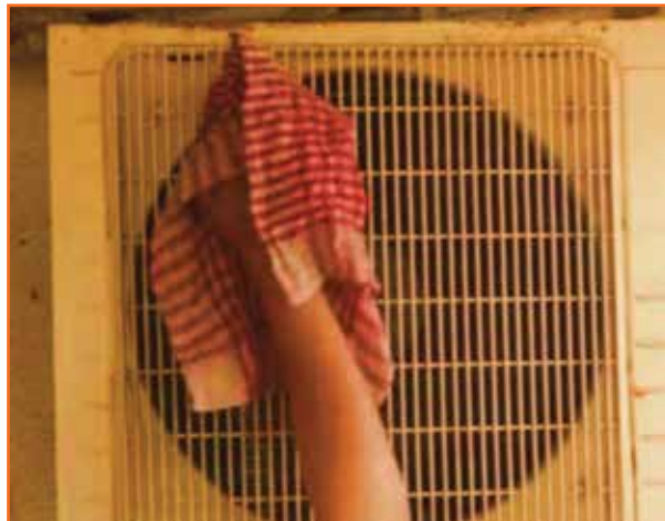
Fig 5.3.29 Cleaning of outdoor unit
