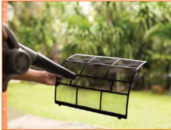
Fig 5.3.28 Washing the filter
