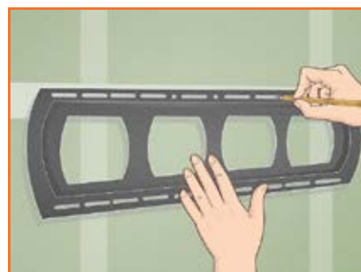
Fig 2.2.14 Marking on wall
