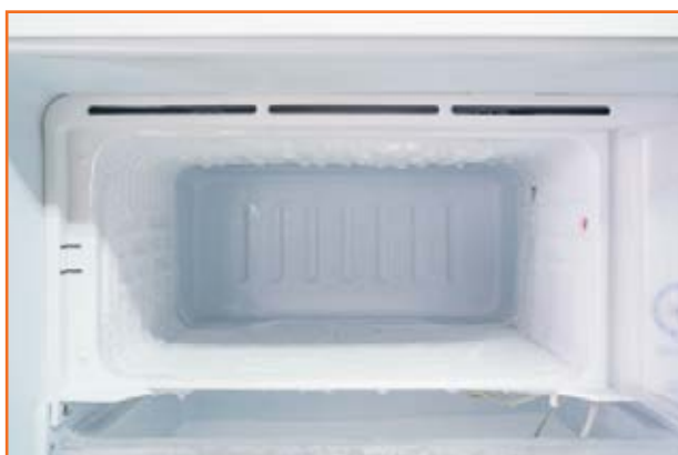
Fig 5.1.15 Frost formation in the freezer of DC refrigerator
