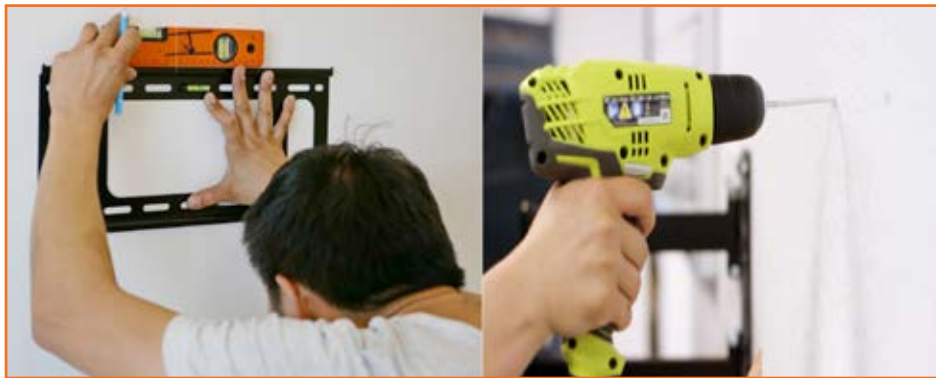
Fig 6.1.13 Marking and drilling holes on wall
